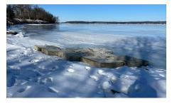
Next, is the work Pierre is doing by helping us get the blocks in place. He has coordinated fabrication and delivery of some new mooring blocks, and has worked with a local surveyor to ensure they are placed according to the anchoring layout provided by StructurMarine. Of key importance is that he will assist during the launch and assembly of the docks. His experience working with the docks at the Shipyard will be an advantage to us.
